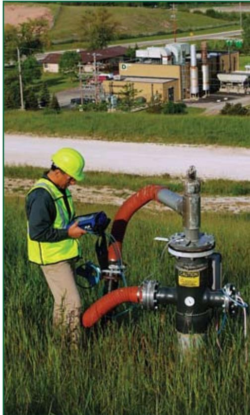
**Methane gas is drawn out of the landfill and converted to energy in the plant.**
