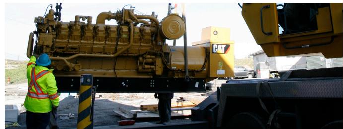
One of five engines arriving at the facility, which will convert landfill gas to electricity.
